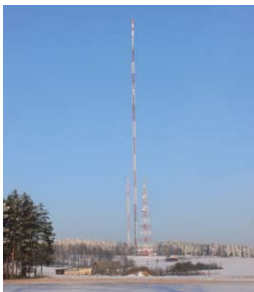
Fig. 51: 300m Tall Tower near Bialystok in Eastern Poland, equipped with instruments for continuous measurements of CO 2 , CH 4 , CO, N 2 O, SF 6 and O 2 /N 2 ratio from five heights. (Photo: M. Heimann)
